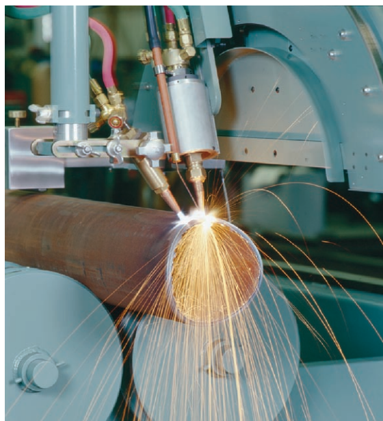
Figure 3. The pipe self-centres in the turning rolls. Only the torch needs to be raised and lowered to accommodate different pipe diameters.
