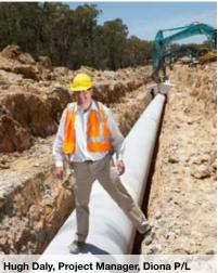
facility. The eight hundred sections of 42" diameter pipe, extending nearly 9kms, slowly takes in gas from the Sydney/Newcastle line over a 24 hour period and compresses it to deliver adequate supply to the gas turbines to be used over a six hour period of peak demand.
