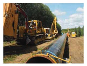
**Figure 2.** The GASTAU pipeline features 34 in. diameter (863 mm), 0.748 in. thick (19 mm) X80-grade pipe and is the first of this grade to be welding robotically in Brazil and the first to use Lincoln Electric's new Pipeliner<sup>®</sup> 80Ni1 welding wire.
