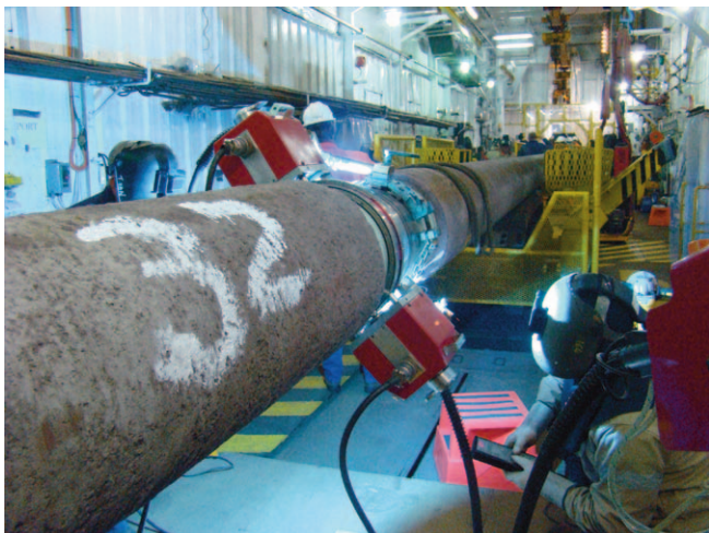
Figure 2. Welding in the pipe tunnel on DB30.
